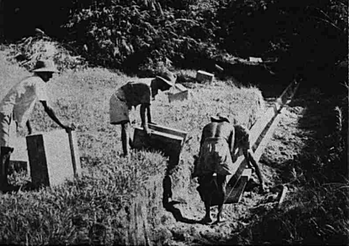
15. Laying anti-malarial drains
