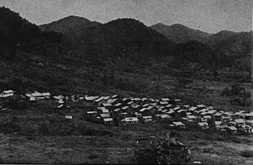
11. New Village in the Bentong Area
